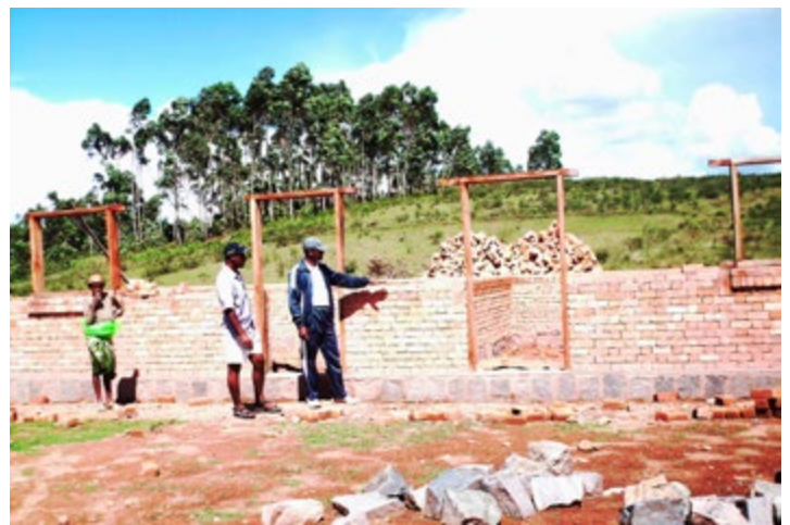
Fig. 3. School construction under progress.
