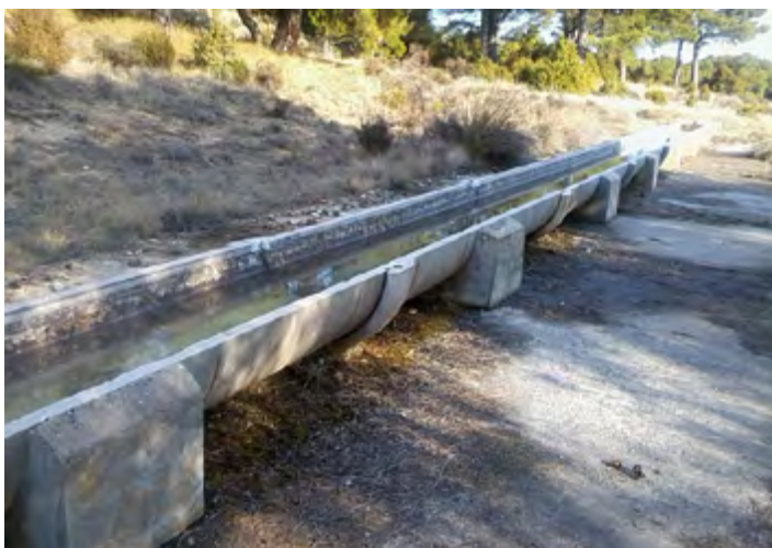
Fig. 3: New water trough made of concrete. Photo: AHE.
