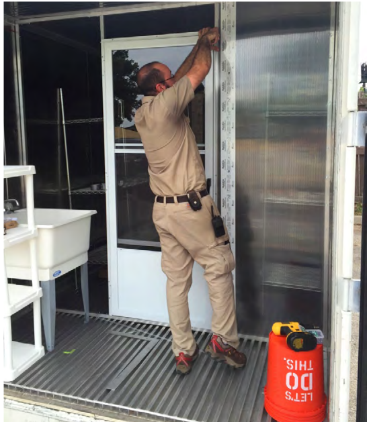
Interior doors are being installed. Photo by: Brandon Greaves.
